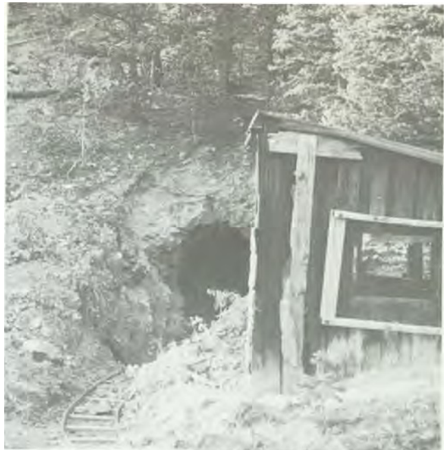
The adit and the shack (the original with some new repairs) of the Golden Chest Mine.
